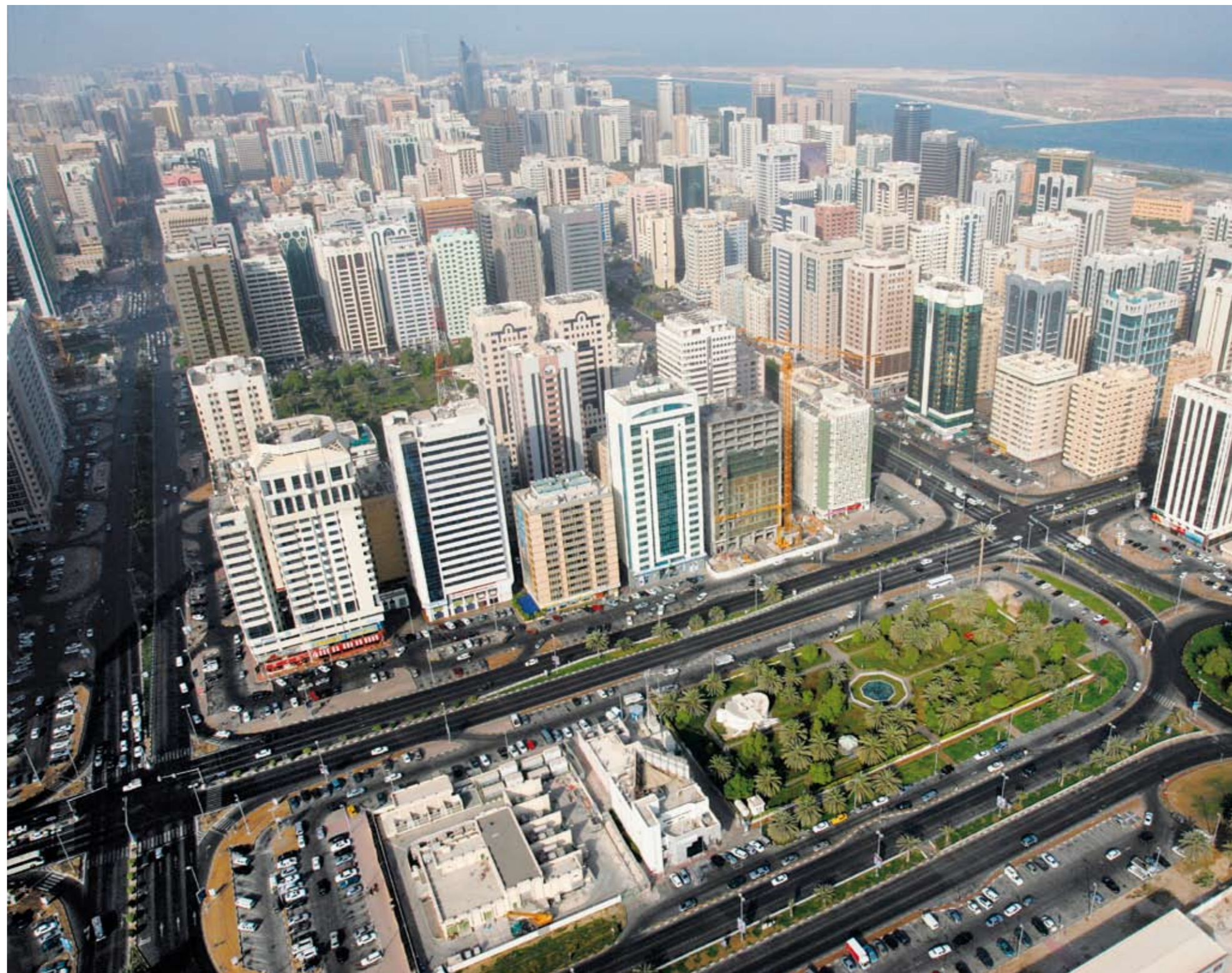
■ Abu Dhabi's transportation and urban master plans aim to create a grid of boulevards instead of large freeways to dissipate
